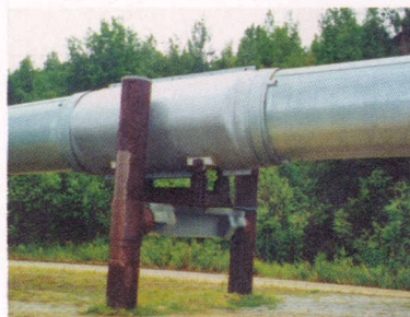
The Alaskan pipeline
